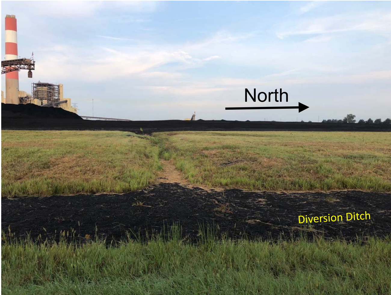
Figure 2 Diversion Ditch Photo September 2021 - Looking West
